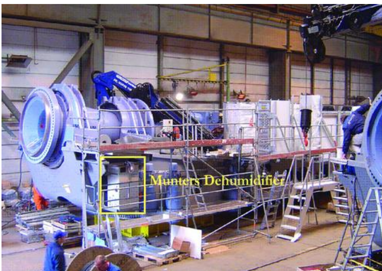
.Installed Munters Dehumidifier
