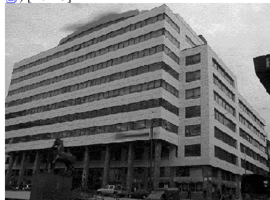
Large Office Building (Portugal) (Leal et al, 2000 [1]) [Ref 17]
