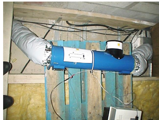
Figure 37 : : Dwelling application after ANA prototype installation
