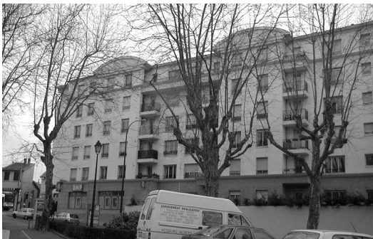
Figure 44: Multifamily building where BIV was tested
