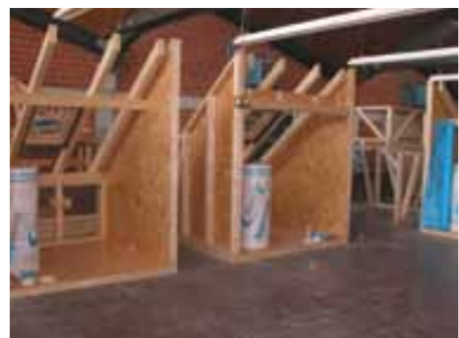
In Germany, we have run a number of training courses for contractors centred on our LDS air tightness system
