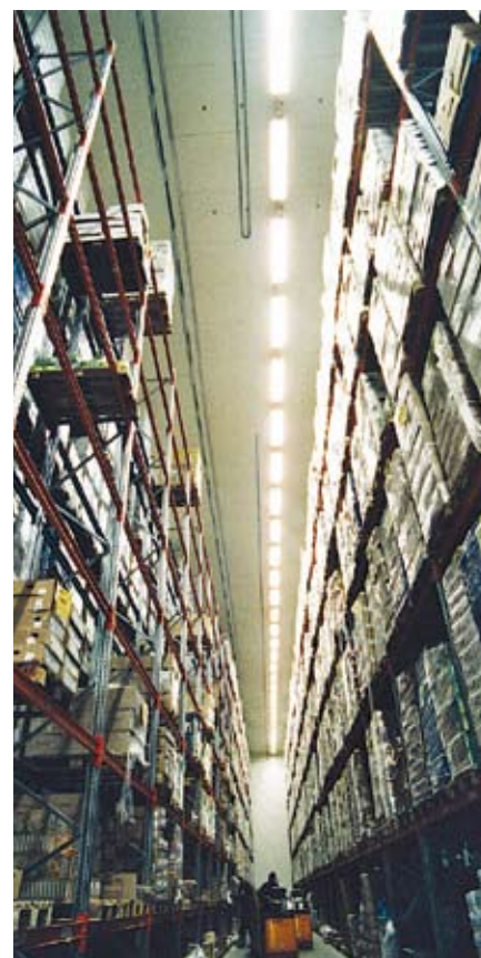
Cold store at Metro's distribution centre in Hamm
