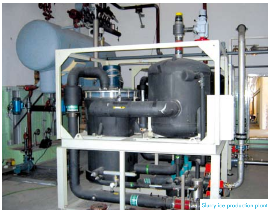
Slurry ice - a mix of ice, coolants and anticorrosives
