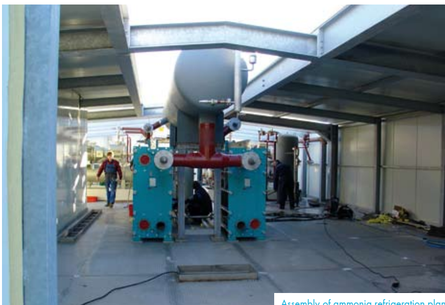
Assembly of ammonia refrigeration plant
