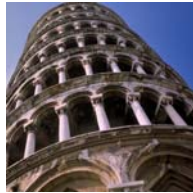
Buildings with static problems
