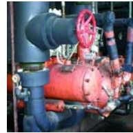
Replacement of existing units
