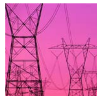
lower electrical output
