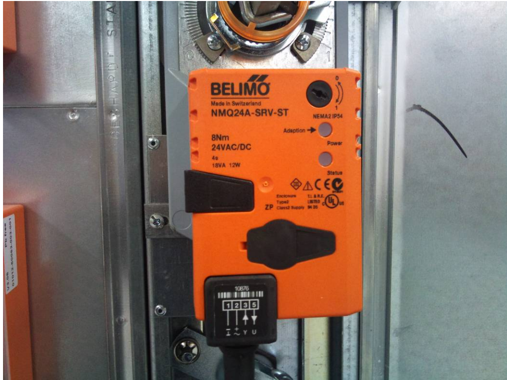
Fig. 8 Drive for louver damper Belimo NMQ24A-RV-ST
