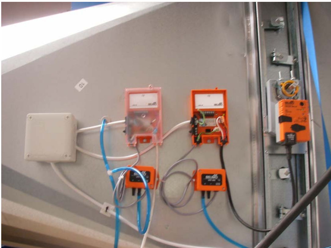
Fig. 11 SAFETY WAY® control components of outlet air unit with louver damper SMAY PWII-S
