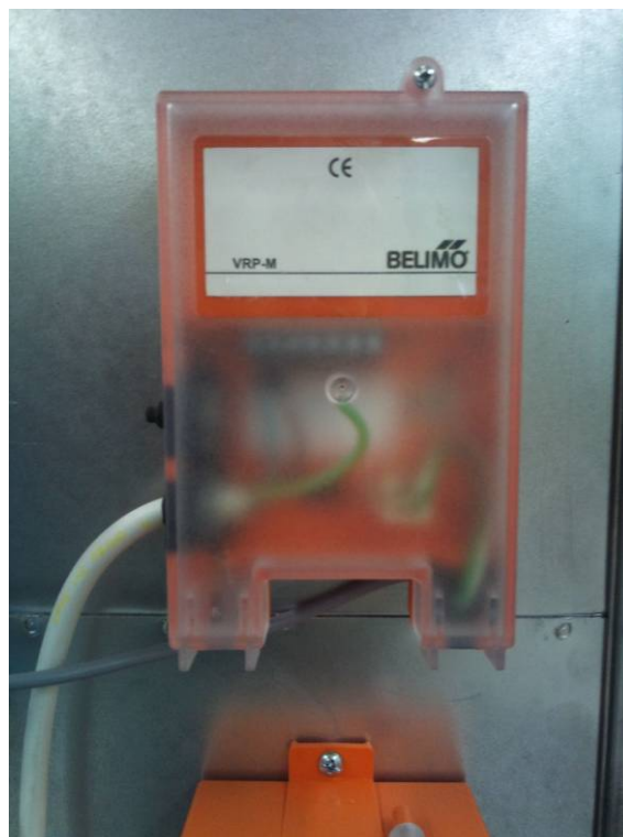
Fig. 6 Belimo VFP300 pressure differential sensor
