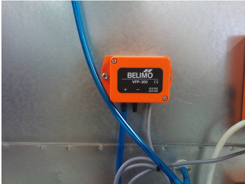
Fig. 6 Belimo VFP300 pressure differential sensor
