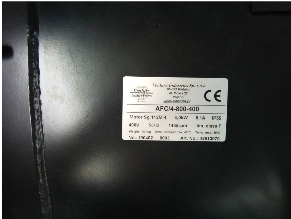
Fig. 3 Fan model plate of supply air
