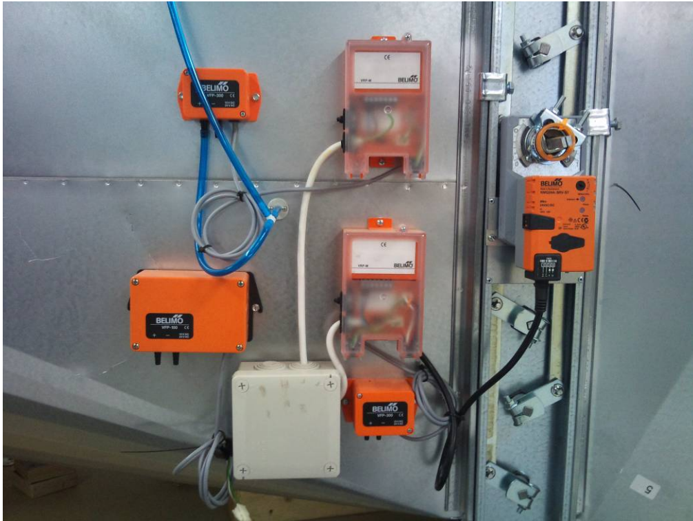
Fig. 5 iSWAY-FC® control components with louver damper SMAY PWII-S
