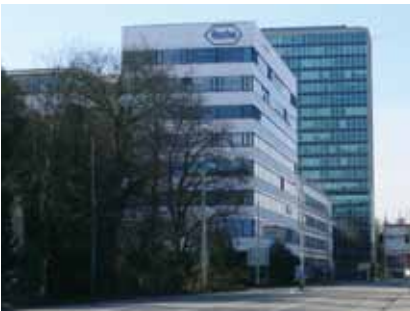
Roche Basel/Switzerland 78 CO-Detectors
