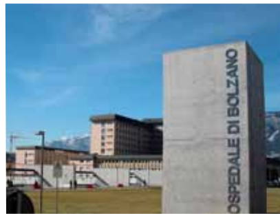
Hospital Bolzano/Italy 64 CO, 64 LPG-Detectors
